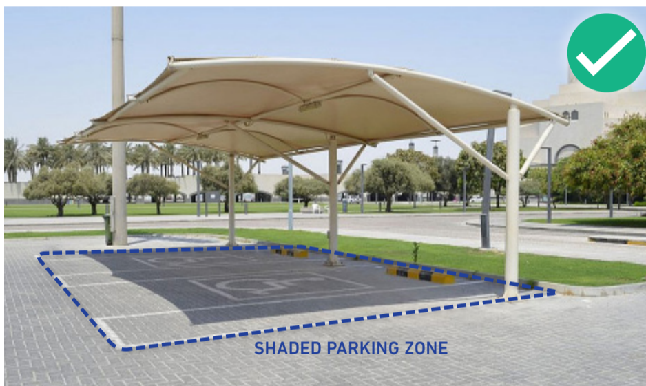
Figure 2.28: Shading provision above Disabled Parking Zones
