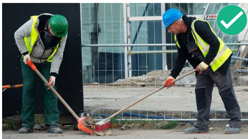
Figure 2.34: Cleaning the site after construction is complete
