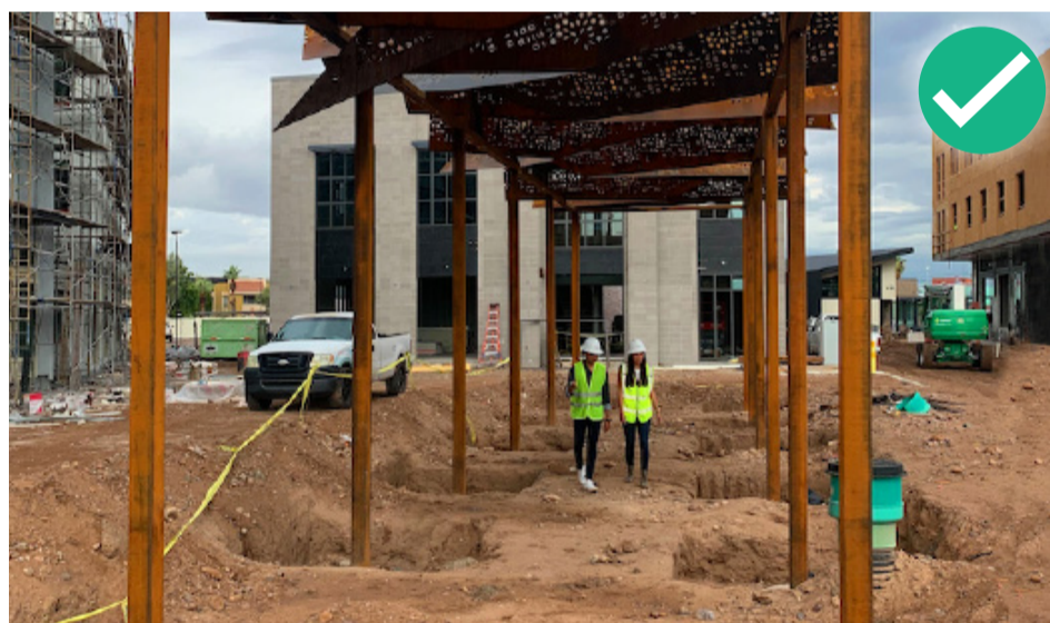
Figure 2.35: Safety Wear (PPE) whilst working on-site
