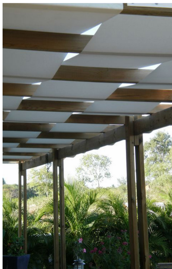
Figure 3.12: Canopy shade of tensile and wooden materials
