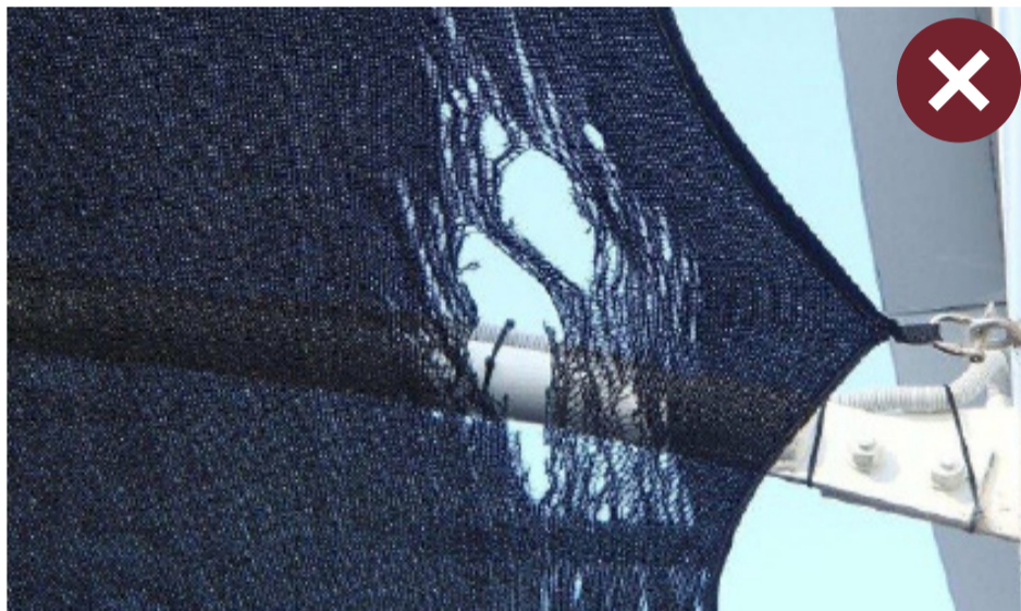
Figure 2.37: Damage to the Fabric Awning Sail
