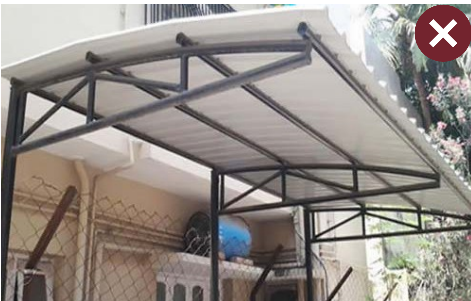
Figure 2.33: Shade coverage made of Prohibited Materials
