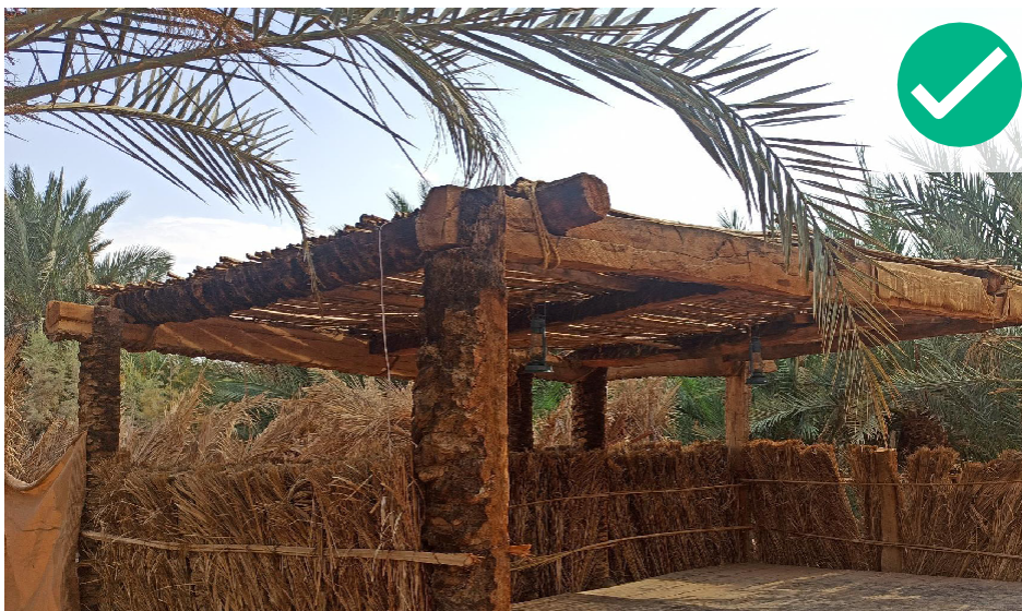
Figure 2.32: Shade Structure made from Recycled Materials
