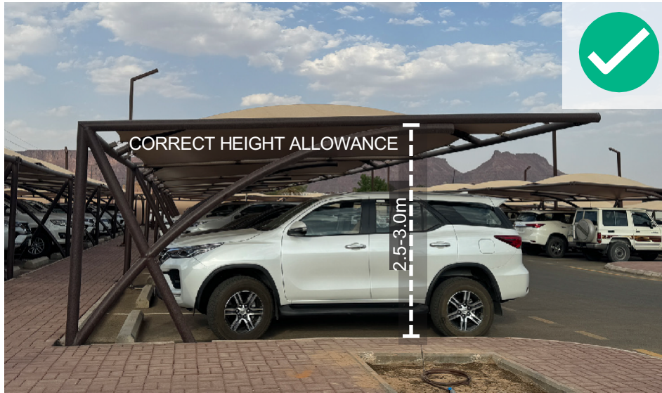
Figure 2.29: Suitable scaled Shade for taller vehicles
