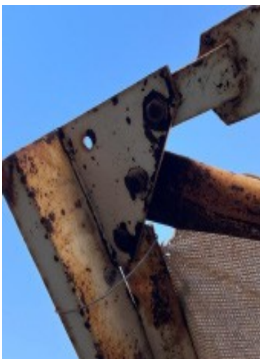
Rust in the hinges of the installation of bridges
