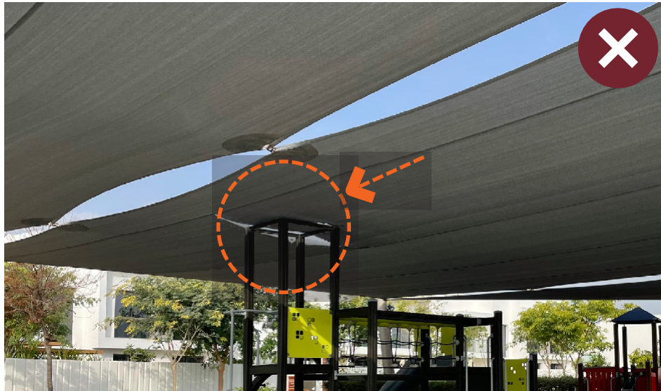
Figure 2.30: Shade Structure too low for purpose
