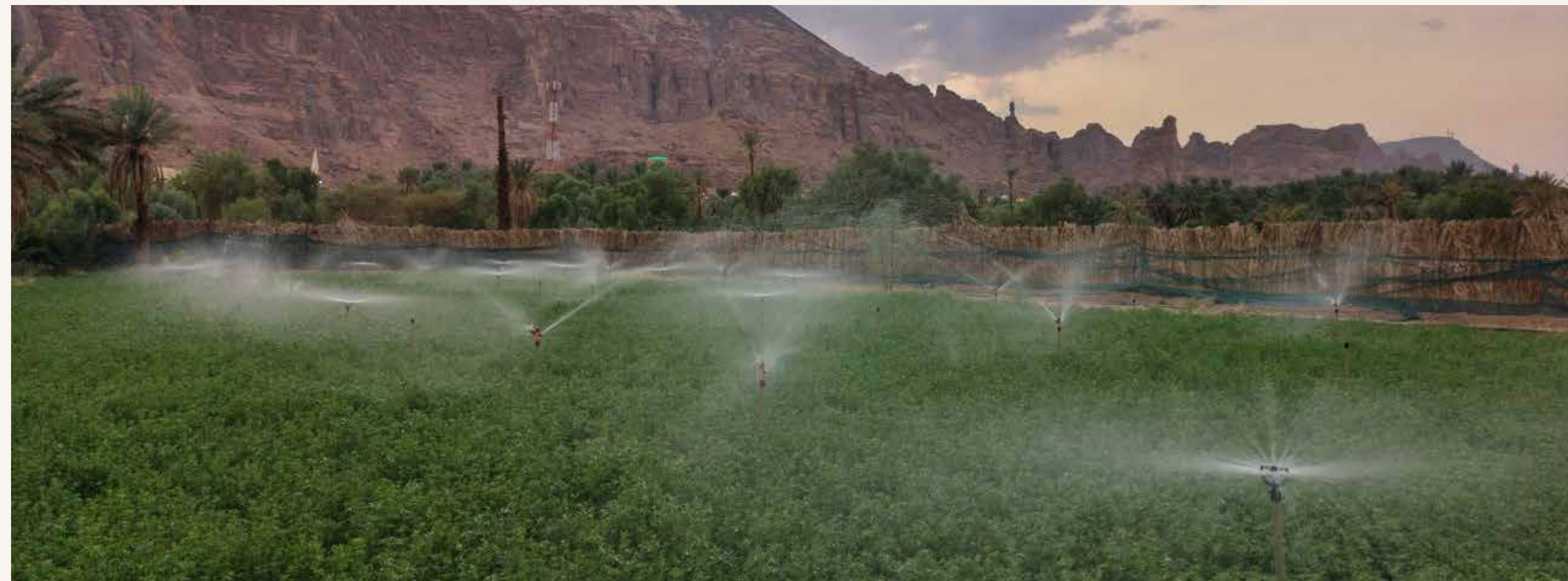
Water irrigation system - AlUla Cultural Oasis
