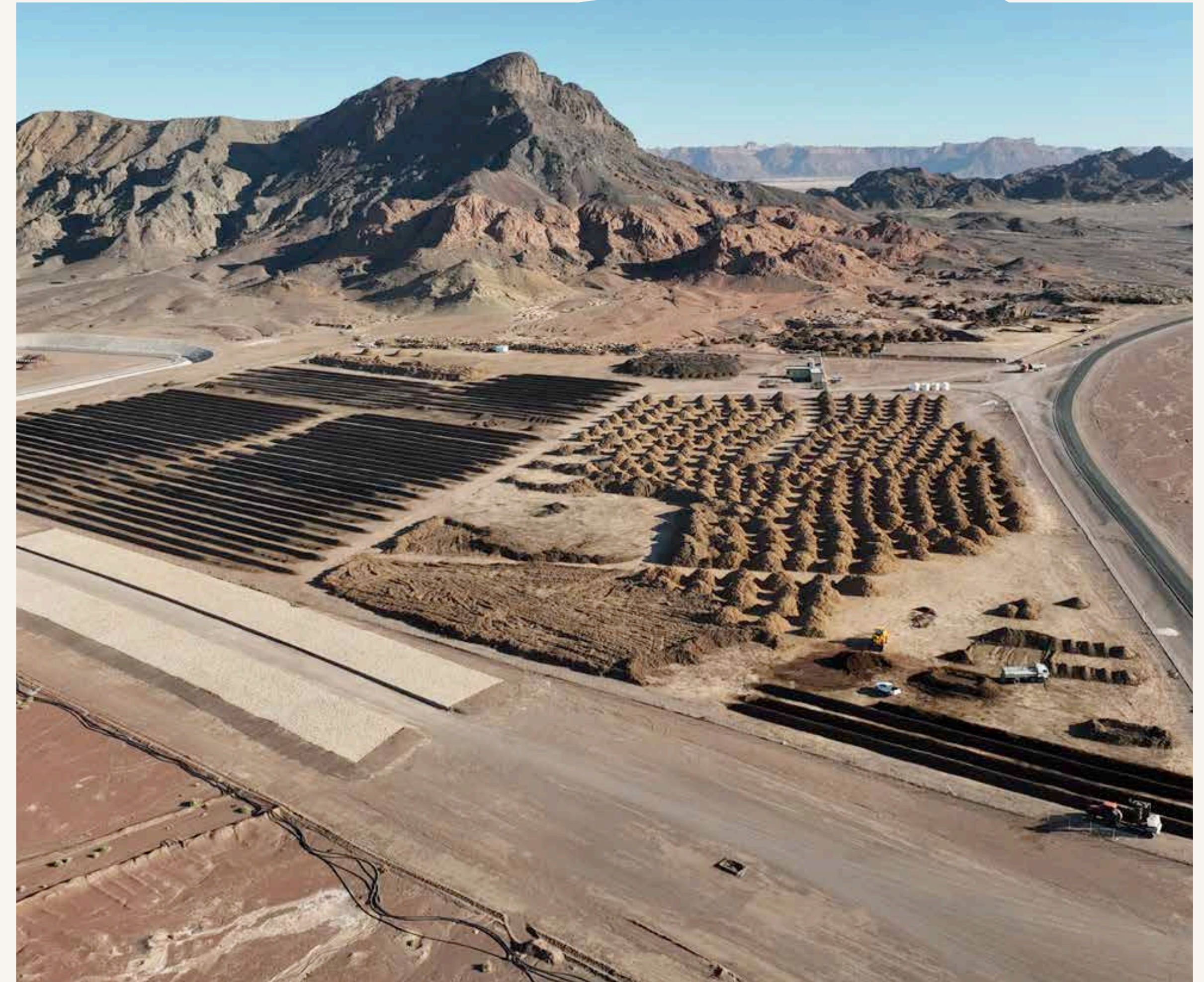
Waste treatment facility - Mughayra
