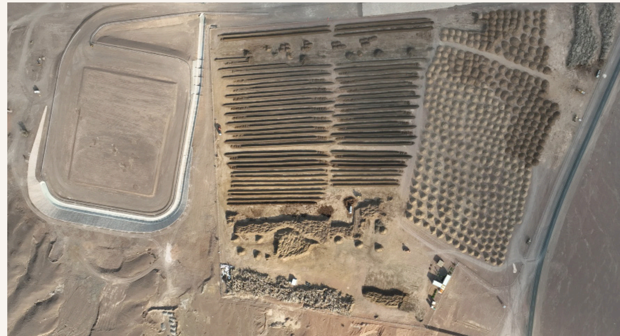
Waste collection site - Mughayra
